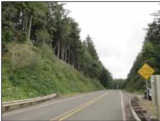
Figure 20. Roadway looking south
