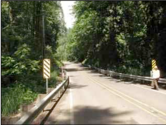
Figure 47. Route 508 looking west
