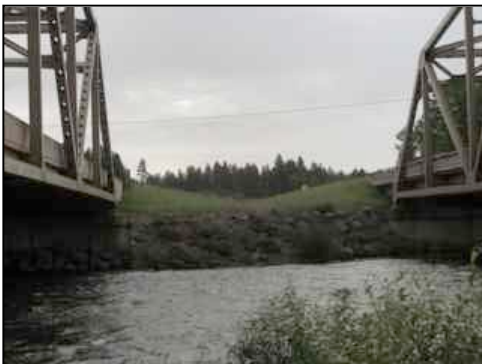
Figure 88. East side median
