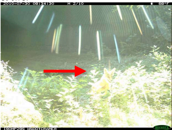
Figure 131. Coyote being repelled from culvert, south entrance, under I-90, mile post 29.
