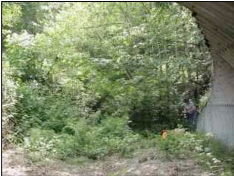
Figure 127. View from north structure outlet
