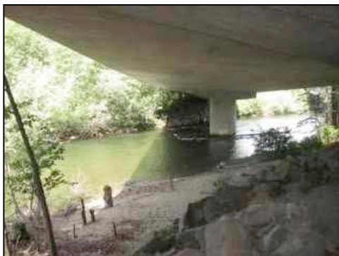
Figure 112. Beneath north structure
