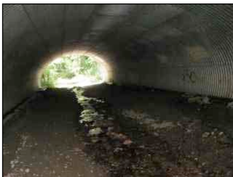
Figure 123. South structure, with unconfined flow
