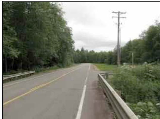
Figure 13. Rte 101 looking South
