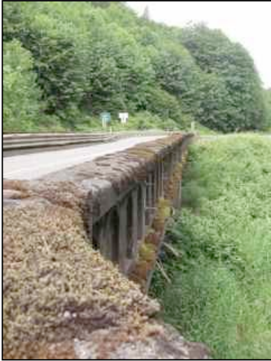
Figure 45. Bridge and adjacent forest
