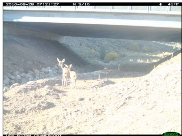
Figure 2. Single span bridge wildlife crossing in Utah, under US 6 © P. Cramer
