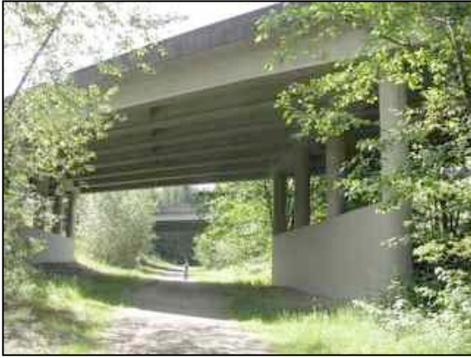
Figure 108. View from north side of slope highway
