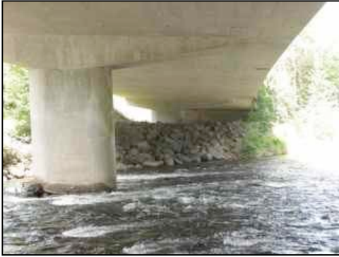
Figure 114. Riprap on west bank
