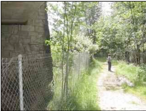
Figure 116. Chain link fencing
