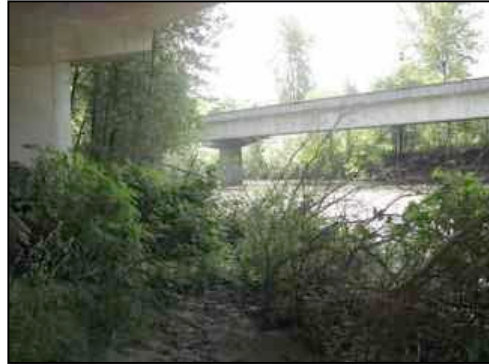
Figure 115. Thick vegetation through median
