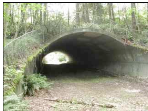
Figure 124. North structure outlet
