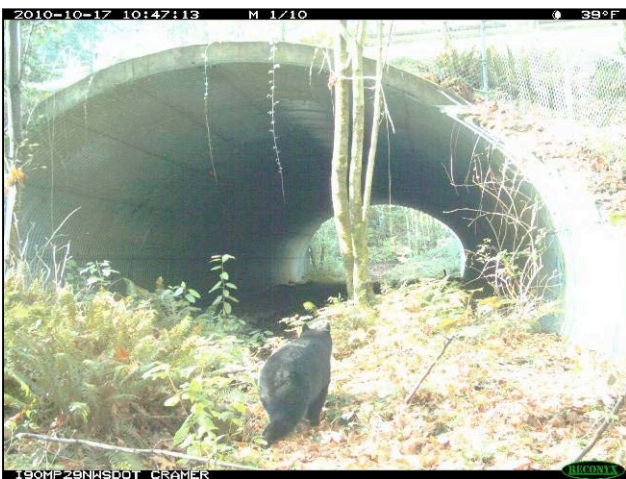
Figure 5. Black bear entering a multi-plate steel arch culvert “game crossing” under I-90 in Washington (built in 1976) © P. Cramer, J. Kintsch, & WSDOT
