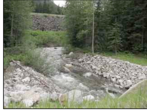
Figure 81. View from north-side structure across median to riprap fill slope along eastbound lanes
