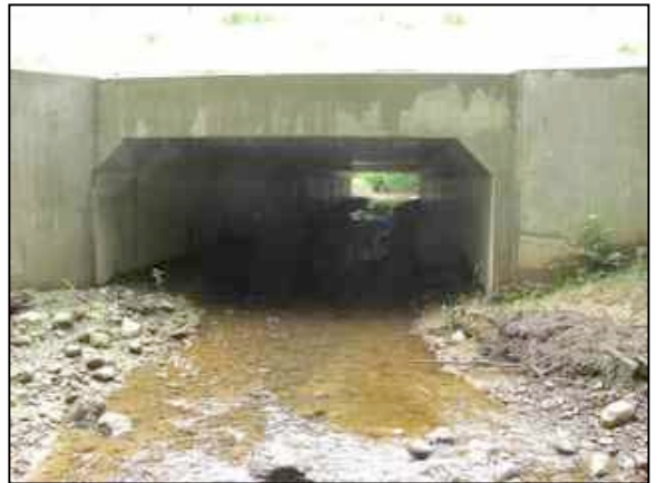
Figure 4. Looking towards outlet
