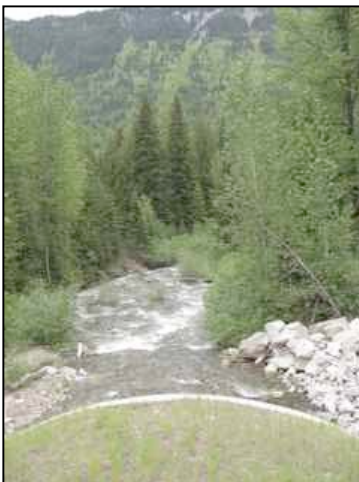
Figure 79. View from north-side structure outlet
