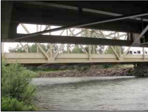
Figure 84. View from beneath south structure
