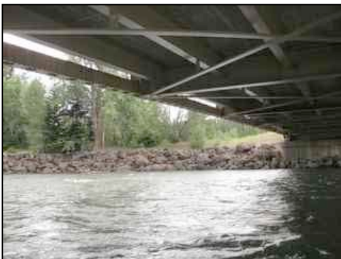
Figure 86. Riprap banks on east side of river
