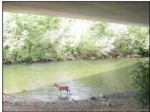
Figure 117. Doe crossing through structure along water's edge
