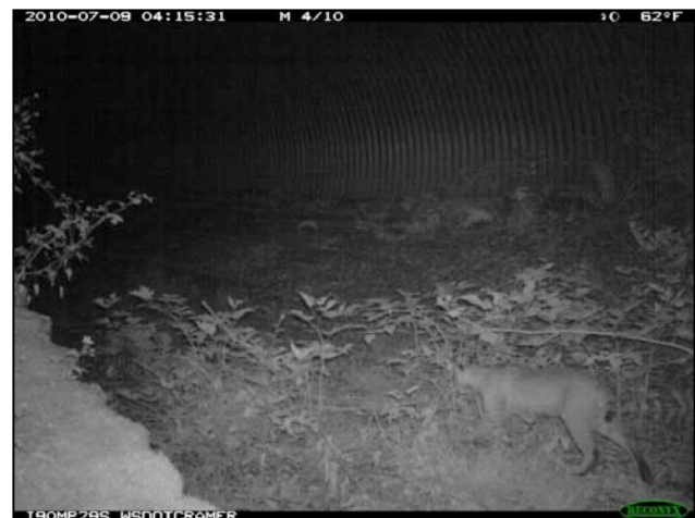
Figure 18. Bobcat using large arch culvert under I-90, Washington © P. Cramer, J. Kintsch & WSDOT.
