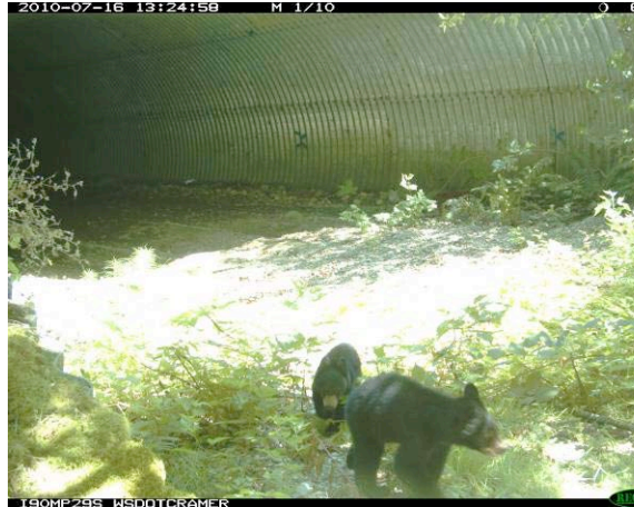
Figure 1300. Black bear cubs following mother through I-90 culvert at mile post 29. Second of two.
