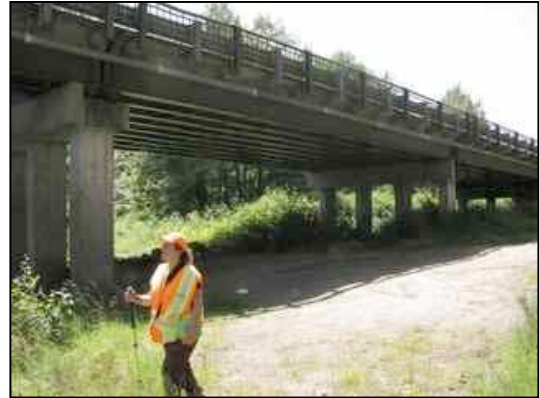
Figure 52. Terrestrial area beneath bridge
