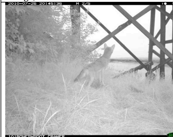
Figure 25. Coyote looking to the west toward Willapa Bay from south end of Bone River Bridge, US 101. Coyotes attempted to move under the bridge at this site, but never appeared to succeed, always coming back.
