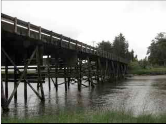
Figure 18. Inlet side, looking west.
