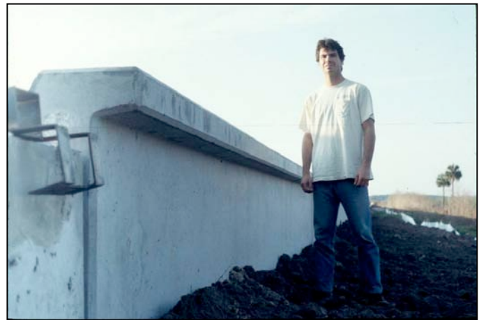
Figure 7. Amphibian and reptile barrier wall at Paynes Prairie State Preserve, along US 441 in Gainesville, Florida © P. Cramer
