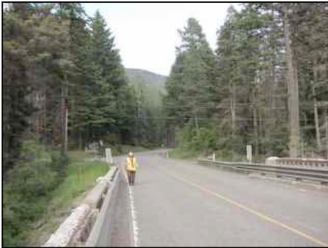
Figure 57. Roadway looking east
