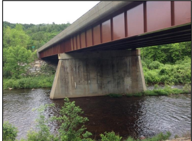
Figure 59. This bridge is classified as “Bridge Adequate” in an AOP survey, leading to an abbreviated survey that does not collect essential information for assessment of terrestrial passage.
