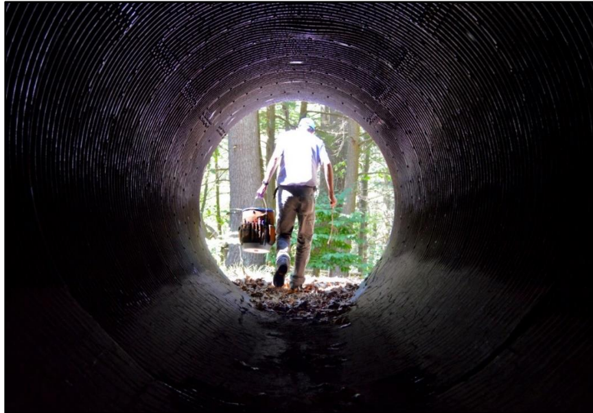
Figure 55. Dry culvert, providing passage for terrestrial wildlife underneath Route 8.
