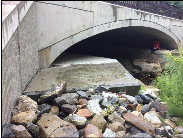
Figure 56. Mixed substrate types of a dry ledge on bridge in Becket, MA.
