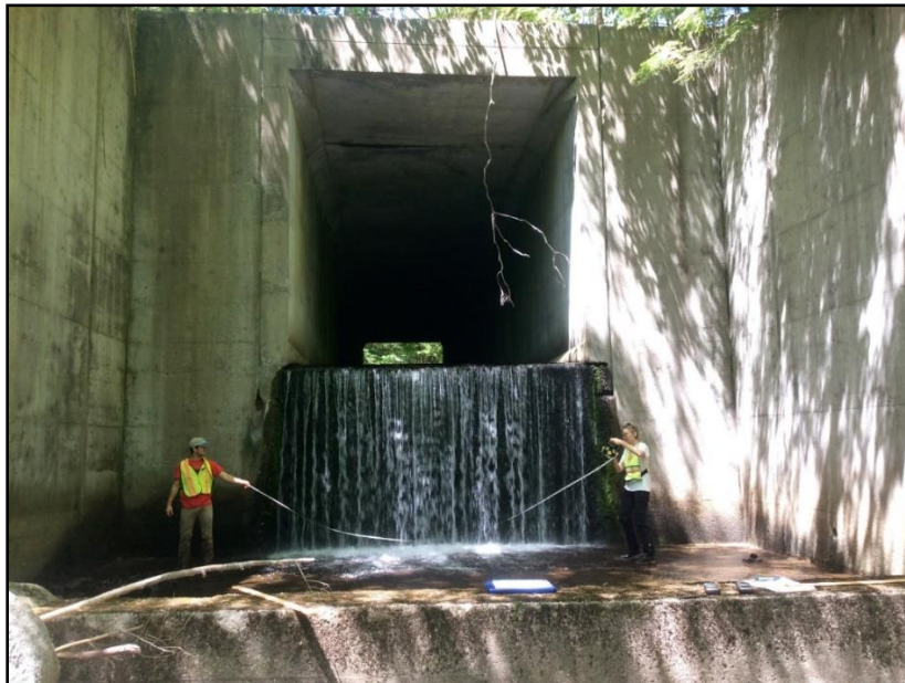
Figure 5. Large box culvert underneath Route 8 near Sandisfield, Massachusetts.
