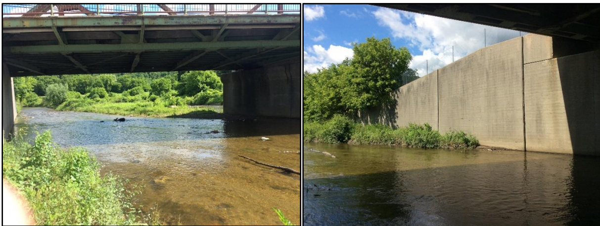
Figure 13. Shallow water in the west cell of this bridge (left) permits dry passage. The approach to this cell (right) funnels wildlife movement along the concrete wingwall on the western side of the bridge.
