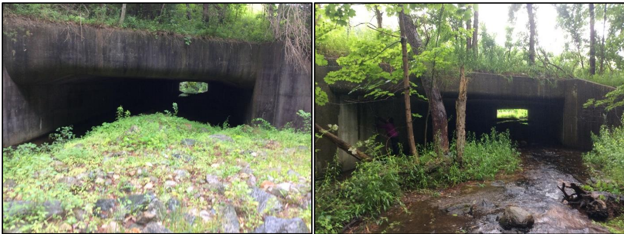
Figure 15. Culvert inlets on I-90 at mile 12.4 (left) and mile 13.7 (right). Although both culverts are large enough to accommodate many species, they differ in many characteristics. The culvert at left received substantially more wildlife activity.
