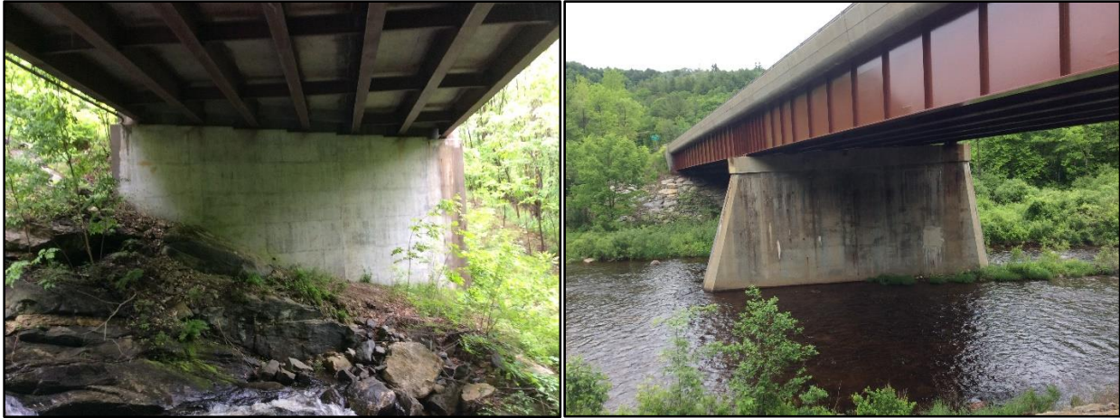
Figure 12. Bridges along Route 8 offering wide banks of dry passage for wildlife. Passage under the bridge at left includes natural substrate, while passage at the bridge at left is along placed riprap.
