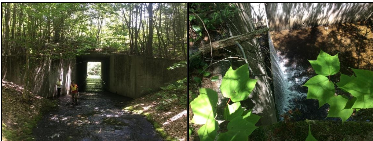
Figure 9. Inlet (left) and outlet (right) at Thorp Brook on Route 8.
