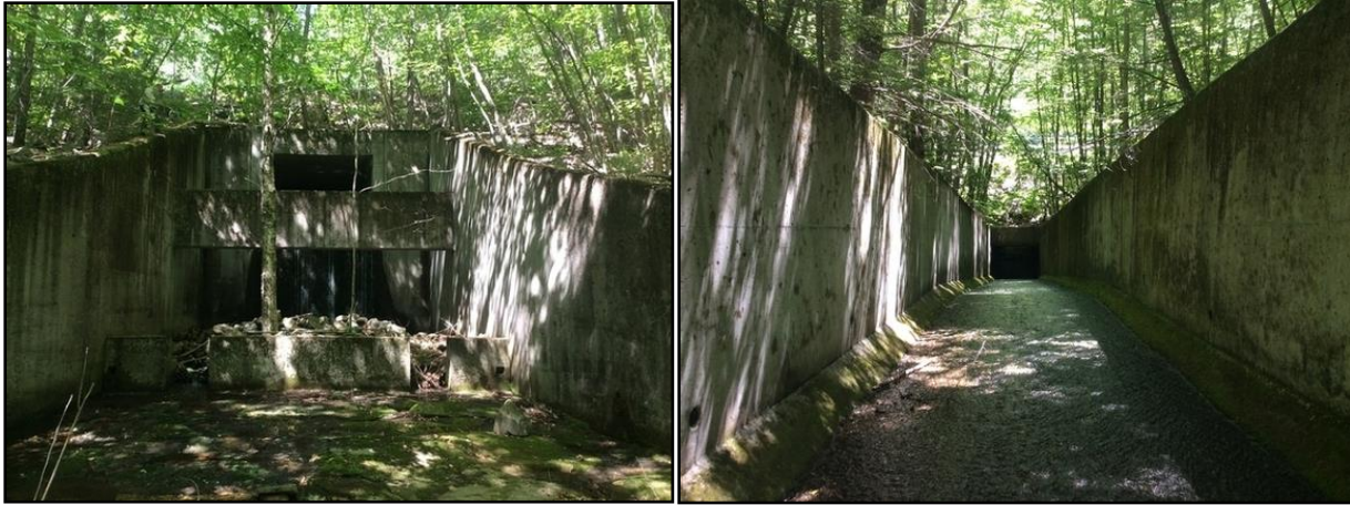
Figure 10. Extensive outlet armoring (left) and chute leading to inlet (right).
