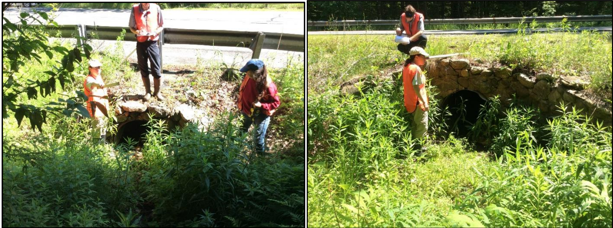
Figure 8. Small culvert along Route 8.
