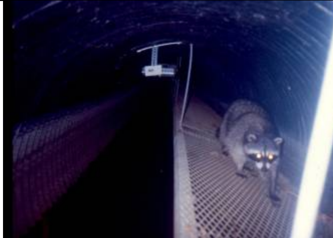
Raccoon using a raised shelf as a dry pathway through a culvert under Highway 93 in Montana ©K. Foresman
