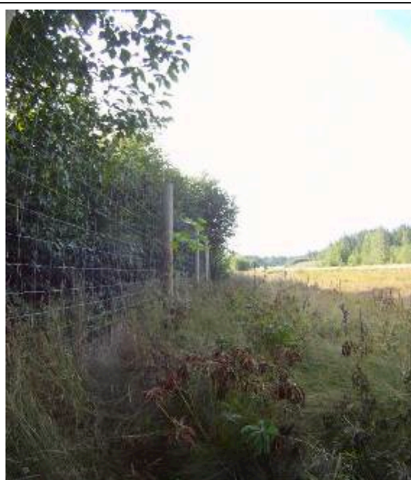
Figure 12: An eight-foot-tall fence-line suitable for excluding ungulates.
