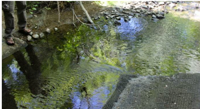
C. Well-lit box culvert, with down-welling light at mid-point
