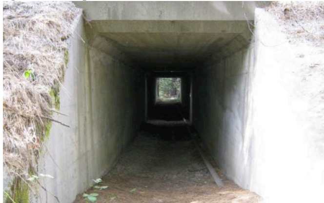
Figure 11: Culvert attributes appropriate for wildlife.
