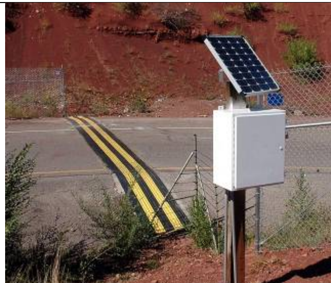
Electro-mat, Electrobraided fencing, 8-foot fence and solar collector on N.M. 333.
